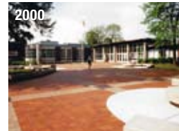
2000 Greenwich High School completed. This was the first joint venture project with O&G Industries. It led to three more ventures worth $200 million.
