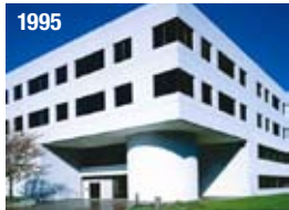
1995 A.P. Construction renovated Hyperion Software's Stamford, CT-based worldwide headquarters.
