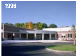
1996 New Canaan's three public elementary schools were completed. This was the largest job for A.P. Construction to-date.
